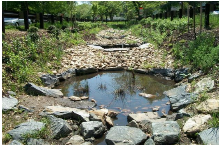
Figure 6.10 Loose Stone Check Dam
