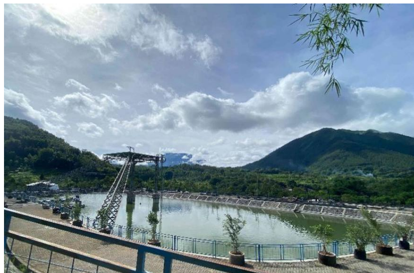
Figure 6.23 Pond Construction Application
